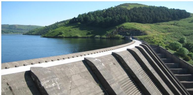
Figure 2. Impoundment Hydroelectric Power Plants (Dam) [17]
