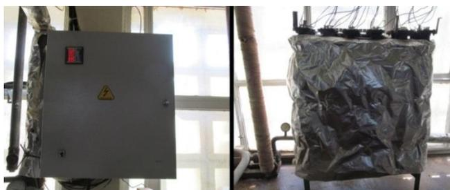
Figure 3. Electrical heater and its control panel.
